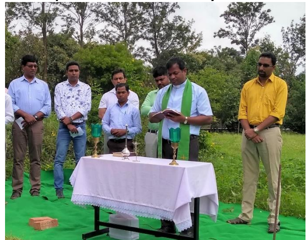
Fr. Sudhir Kujur leads a prayer for the laying of the foundation stone.
