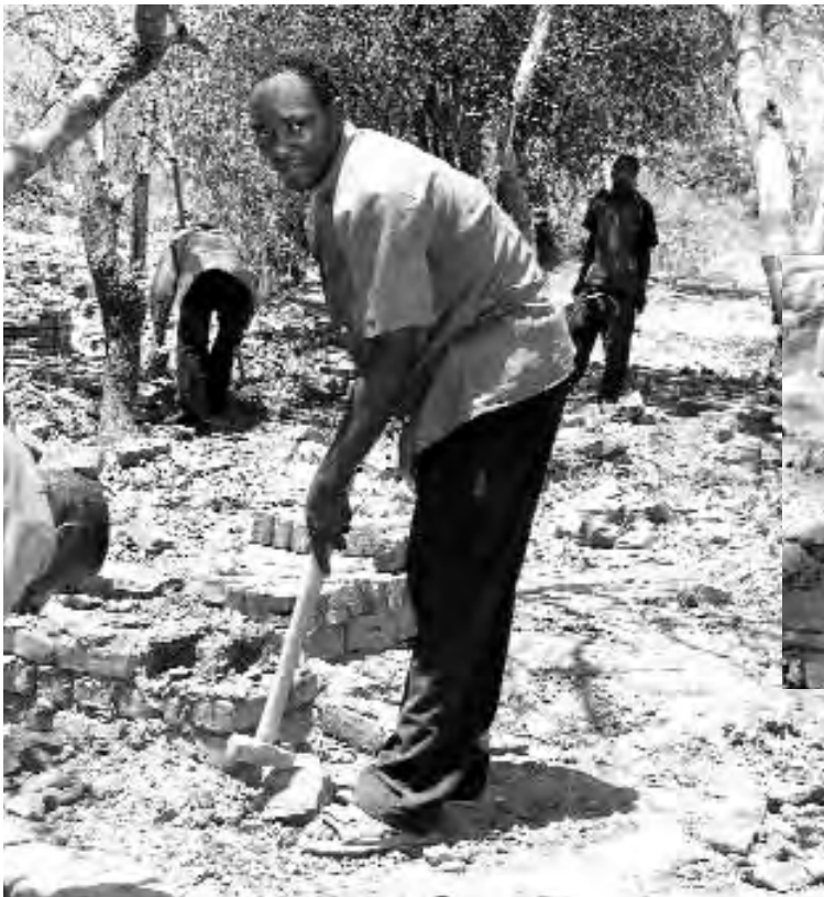
Students practice bricklaying as part of their vocational training.
